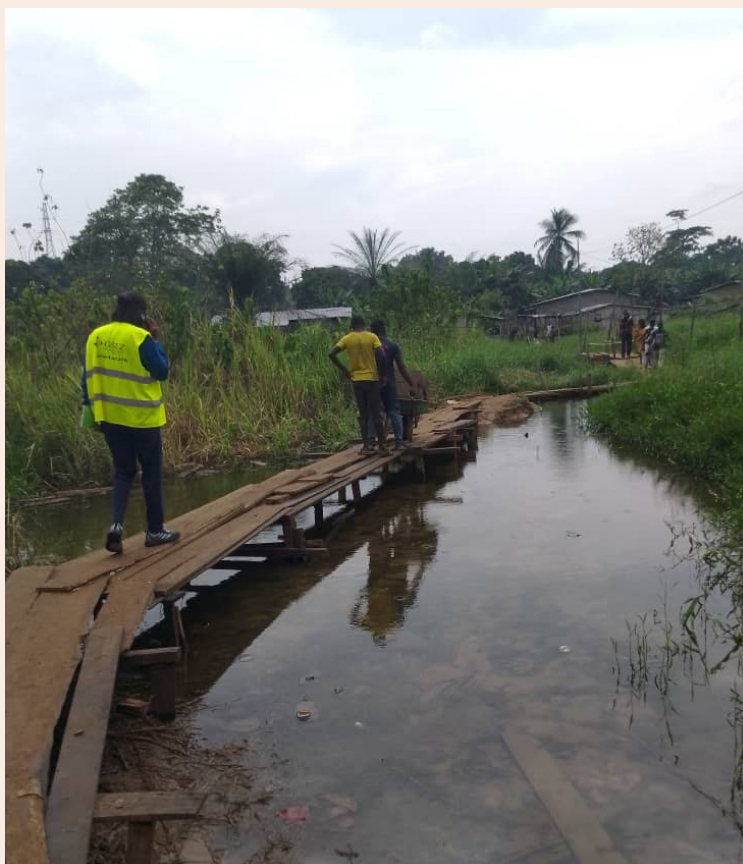
Bridge under construction to ensure safe access for school students in Gabon.
